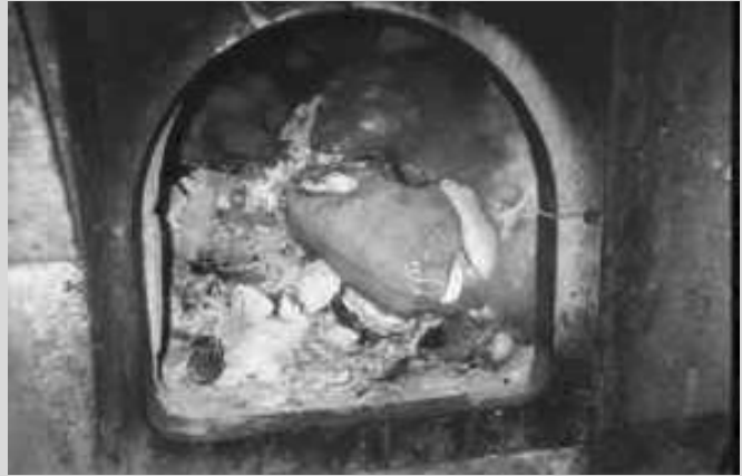
Burning unsorted waste at on-site incinerator in Ngelwezane Hospital, South Africa © groundWork
