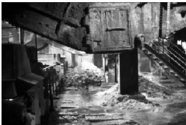
Bottom ash from furnaces and fly ash that fell from the electrostatic precipitators at the Harrisburg incinerator in Pennsylvania.
